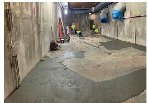
Tunnel after air handlers removed and floor drains replaced.
